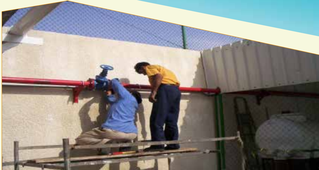
Bypass valve installation
