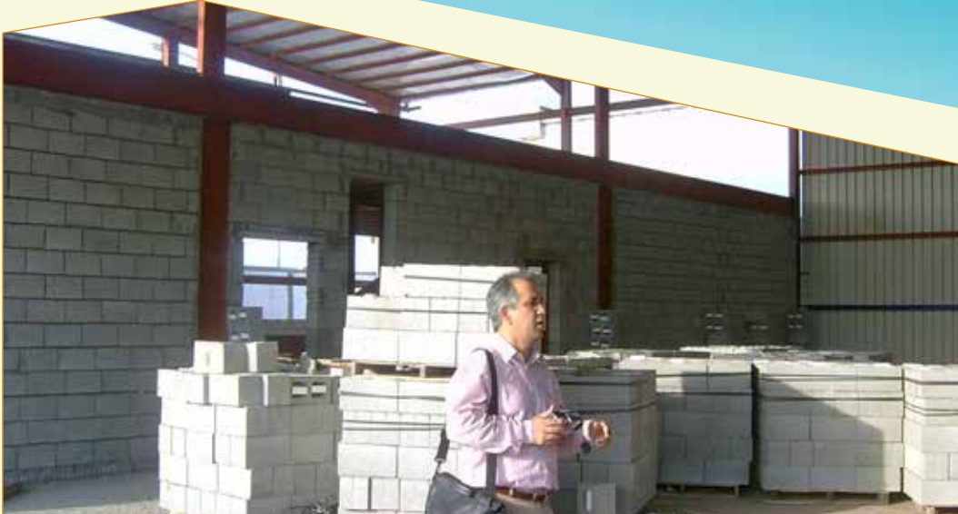
Inspection by the GM
