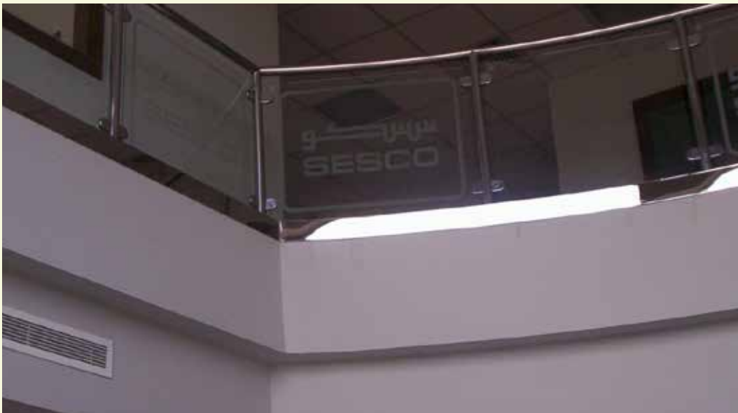
Stainless steel railing work
