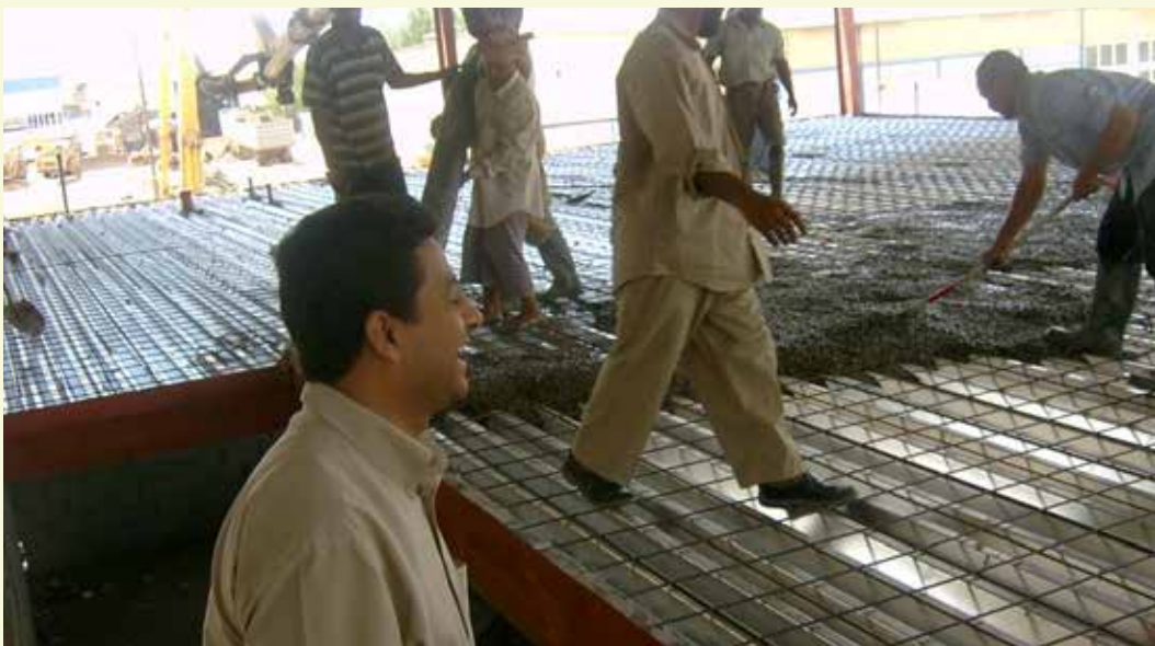
Casting of Mezanine Floor
