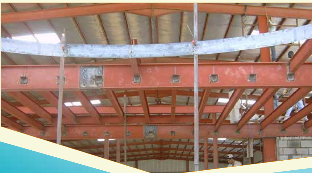
Steel structure Atrium Area
