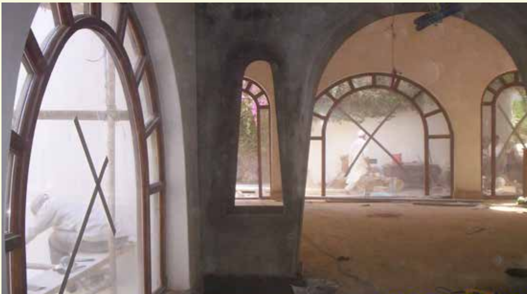
Wood work and Benjamin floor tiling
